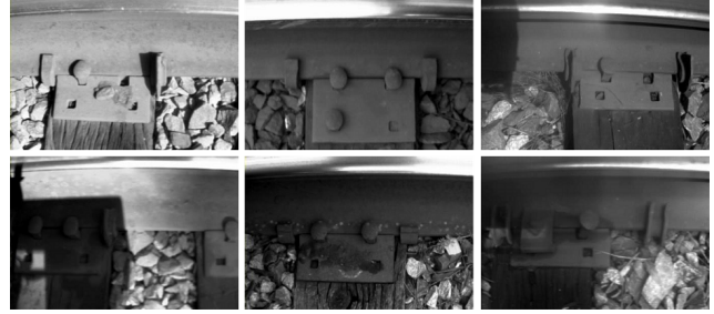
Figure 5. Anchor appearance has a high variability coming from diversities in anchor type, size, shape, camera view point, occlusion and light condition.
